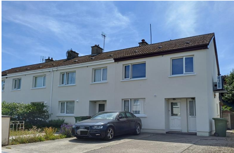
Energy Retrofit works completed at Seamount Drive Kilcoole 2025.
